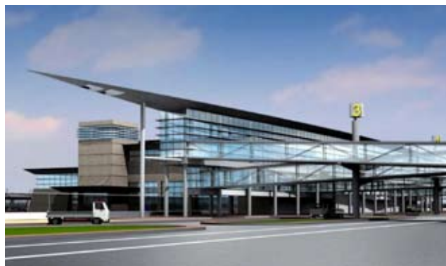
A view of the Borg El Arab Egyptian airport.
