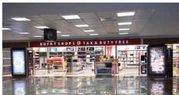
1,328 m 2 will be renovated.
