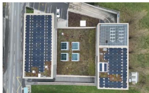
View from above: our photovoltaic unit on the roof of the bank branch building in Eschen
